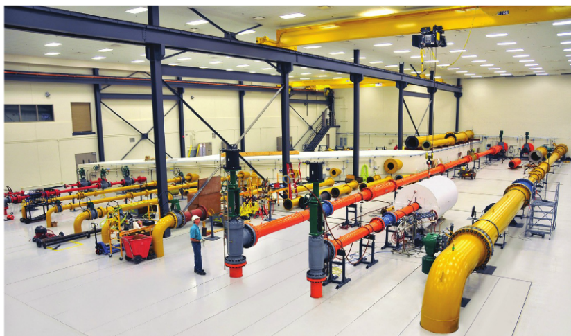
□ The 26,900-square-foot (2,500-square-meter) flow lab in the Emerson Innovation Center
