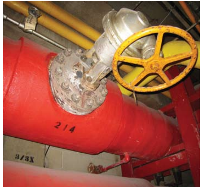
Wedgeplug installation at Chicago's O'Hare Airport. O-ring style plug used to supply water to the airport and also used in hot water loop to melt ice on runways.
