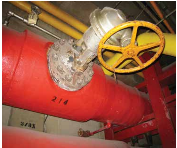
Wedgeplug installation at Chicago's O'Hare Airport. O-ring style plug used to supply water to the airport and also used in hot water loop to melt ice on runways.
