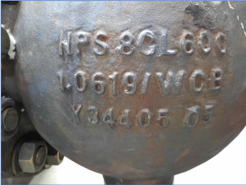
Photo 1: Valve marking and tagging
