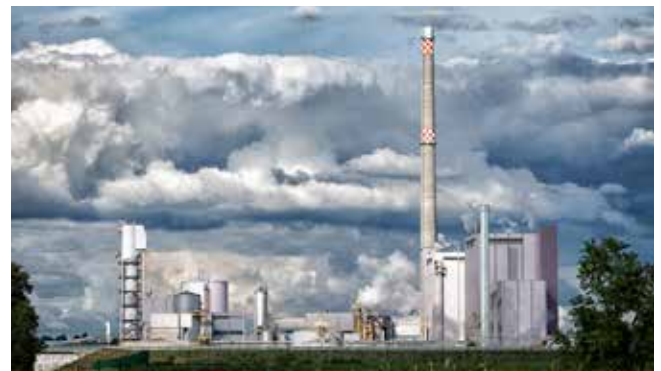
Sugar plant Centerline RS installed in a thin juice station
