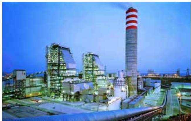
Power Plant Iskenderun, Seawater FDG (Turkey)
