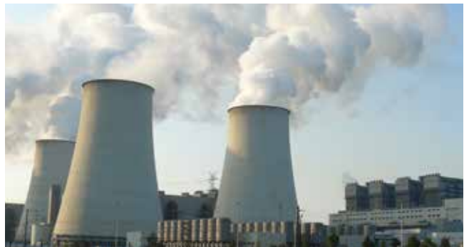
Power Plant Jaenschwalde (Germany)
